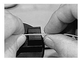
**4.2** Grasp the coated fiber about .25 inches (6 mm) from the bare glass and move the fiber end onto the fiber alignment guide on the assembly tool such that the end is resting on the alignment guide outside of the splice.
