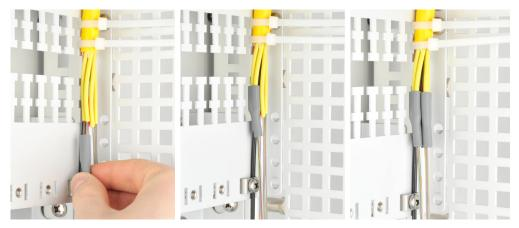
**NOTE:** Depending on the cable profile, different grommets can be used. To install proper one please refer to the table on the bottom of this page.
