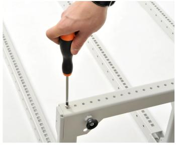
**1.6** Mount upper profile on the opposite side of the rack and tighten all screws.
